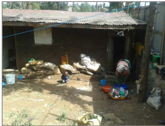
Sand filled sacks piled as a flood protection in Repi
