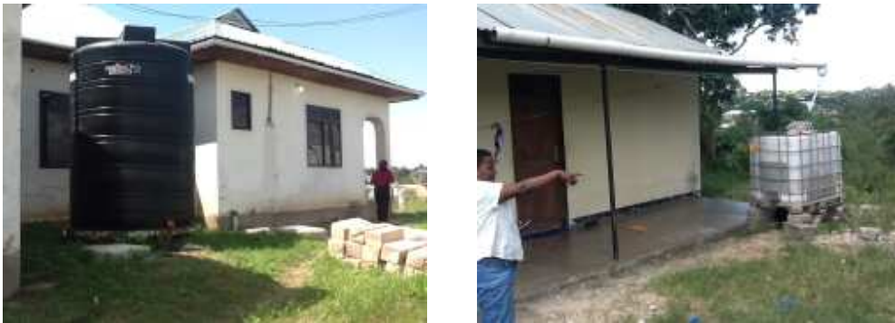
Figure 5: Rain water harvesting systems at house level at Mbezi Luis sub-ward (Upstream)
